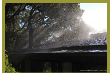
Photo 1. Roof mounted sprinkler.
